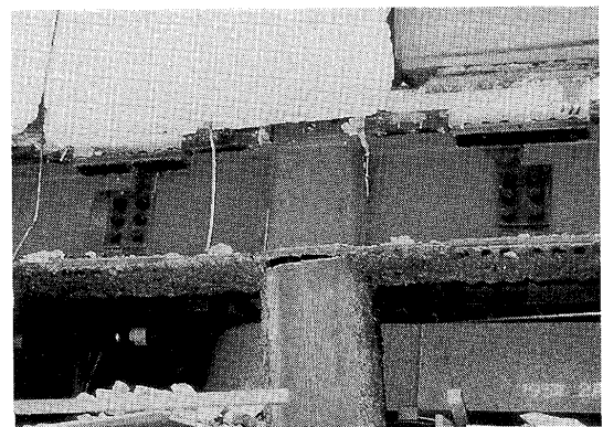
Fig. 11 Crack and fracture probably caused by insufficiency of strength. 6)
