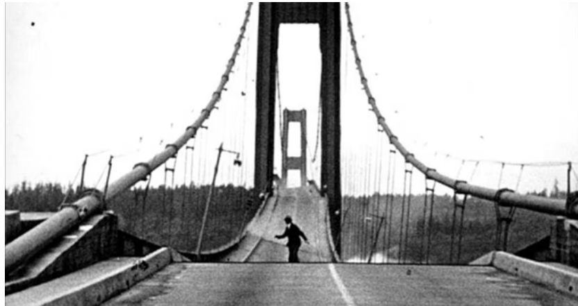
Figure 1-13 Collapse of the Tacoma Narrows Bridge [50]
