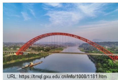
(h) Pingnan Third Bridge (2020)
