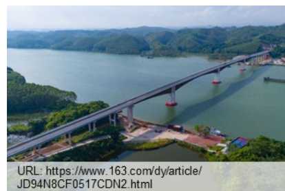
(j) Feilong Bridge (2024)
