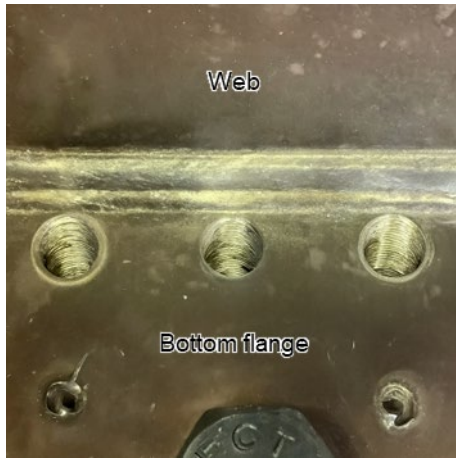
(b) Drilling holes
