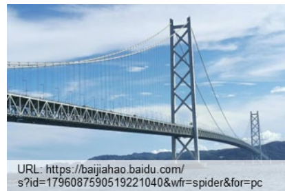
(f) Akashi Kaikyo Bridge (1998)
