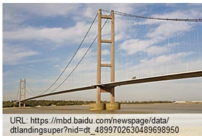
(e) Humber Bridge (1981)
