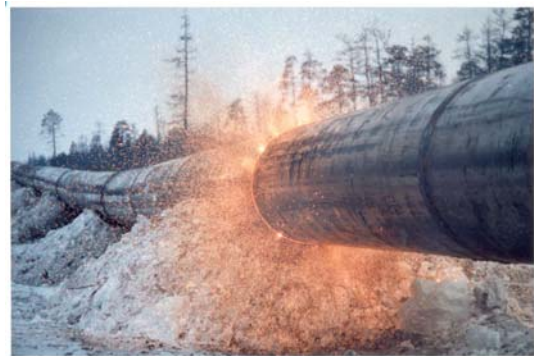
Fig.13 Flash Butt welding in Siberia.
