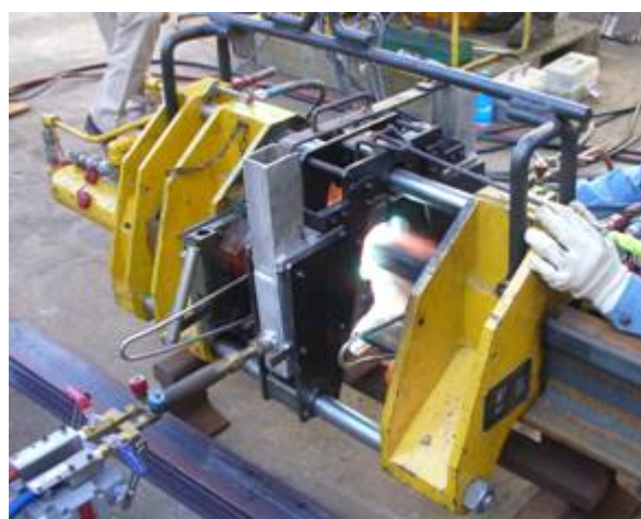
Fig.4-13 Gas pressure welding of rail
