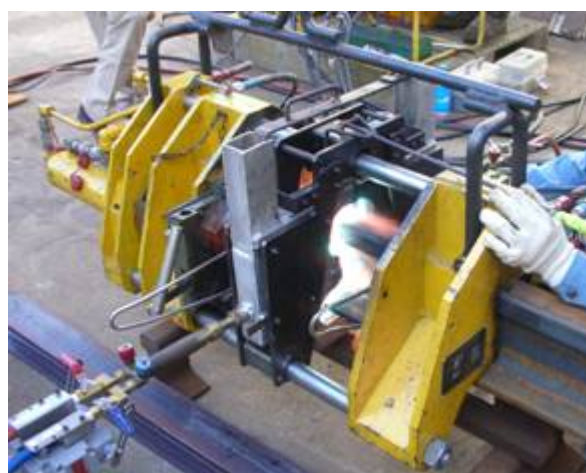
Fig.4-13 Gas pressure welding of rail
