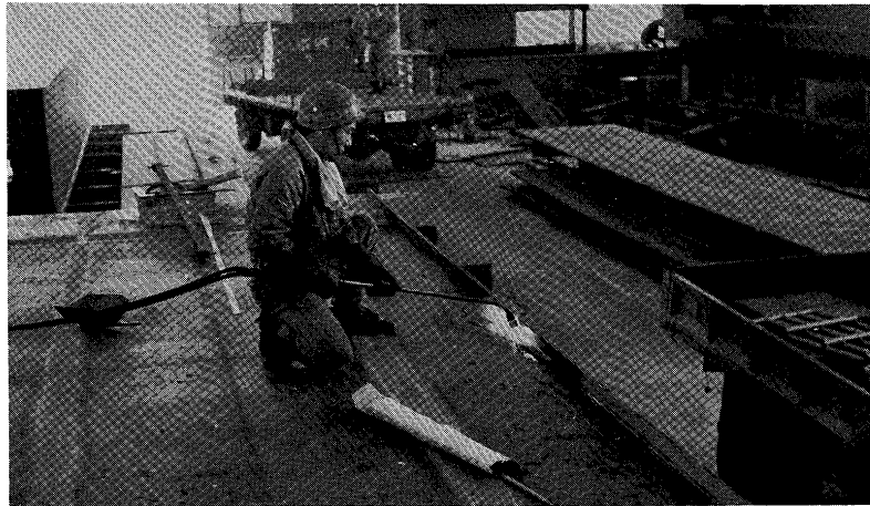
Photo. 1. Preheating work using single nozzle gas torch.
