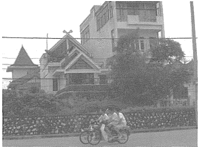
Figure 7. Housing in Au Co Road House
