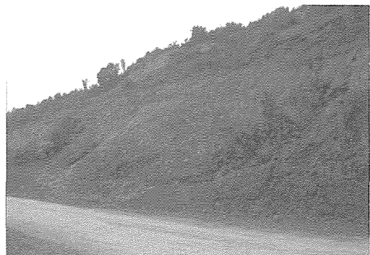
Photo 3.8. Landslide block composited form shattered rock
