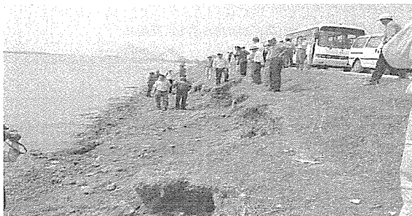
Figure 3. 650m of central seadyke in Tan Boi village, Thai Do commune, Thai Thuy district, Thai Binh province eroded due to storm Damrey (No 7) as a result of mangrove absence
