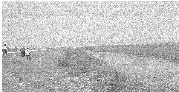
Figure 4. 5km of seadyke protected by mangroves in Thai Do commune and therefore, not eroded in presence of the storm Damrey
