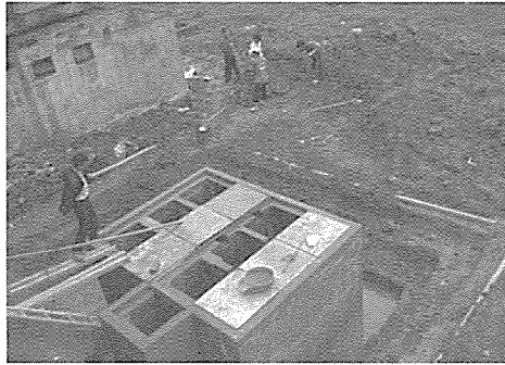
Picture 1. BASTAF implemented in PC building, Ta Thanh Oai commune, Thanh Tri Dist., Hanoi
