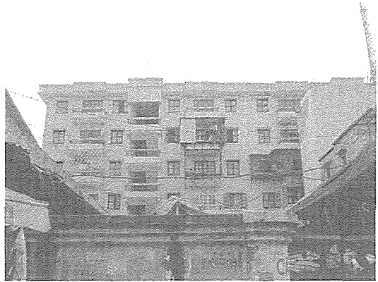
Photo 6. Rebuilding of apartments
