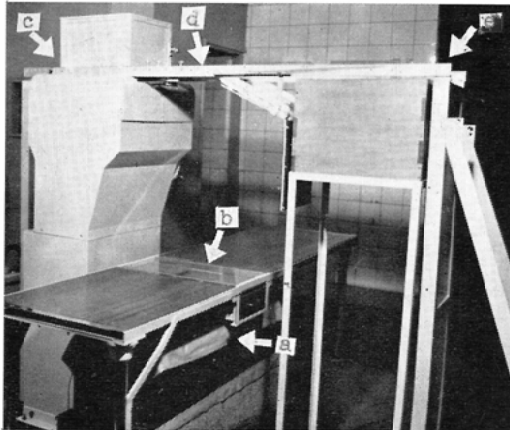
Fig. 6. Film cassette changer for enlargement angiography.
