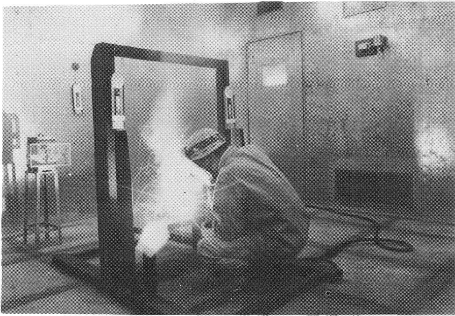
Fig. 2.1 Welding of test specimen in controlled humidity chamber
