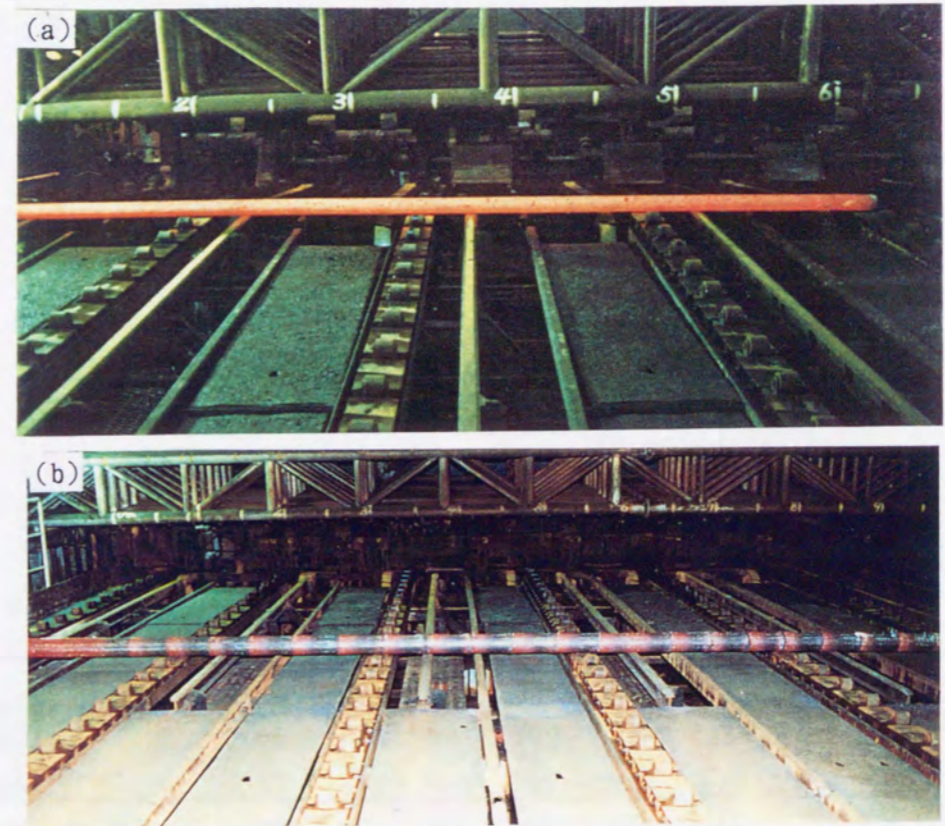
(a)no obvious defects (b)cracks in logitudinal direction
