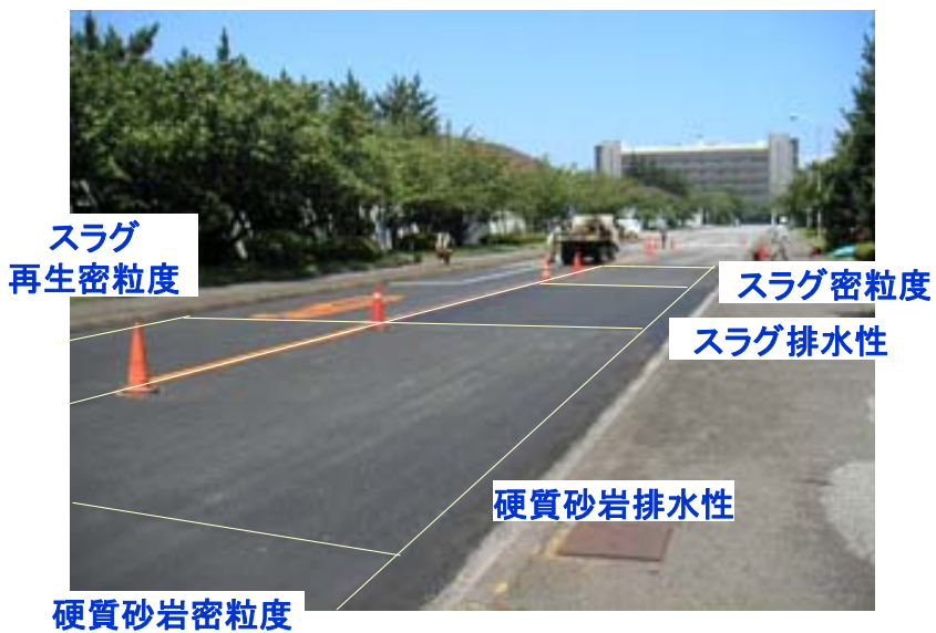
Fig.2-53. View of test pavements after construction.
