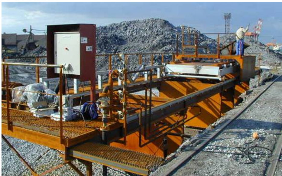
Fig. 2-14. View of pilot plant for slag solidification process.
