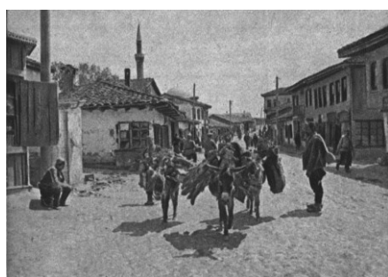
Photo 2 Road towards the SE Gate
