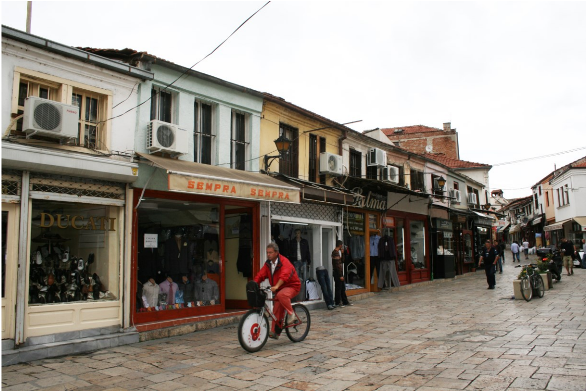
Photo 16 A group of type B units in one building on Street Podgragje in Skopje's Bazaar - Photo by the author
