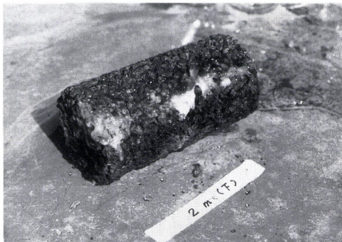
Photo 4. Attached biomass grown on the porous concrete.
