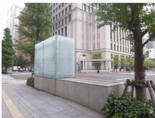
Ventilation / Fire Exhaust
