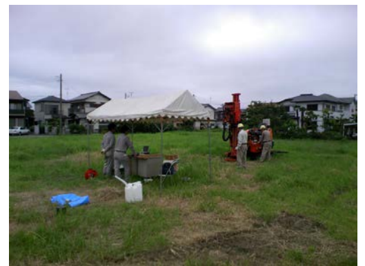
Fig. 4.13 CPT at site
