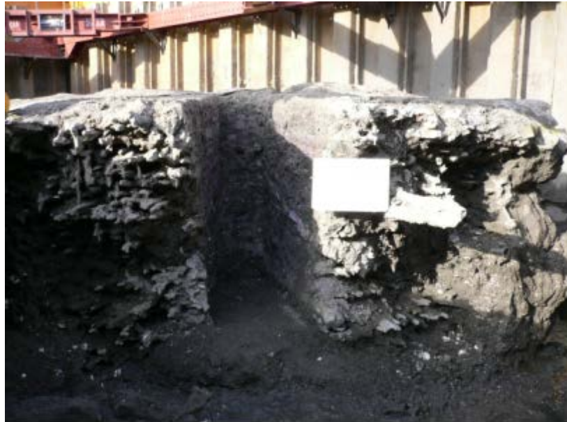
Fig. 4.21 Type 1 : JETCRETE column by the nozzle with flow conditioner with stepped rifting
