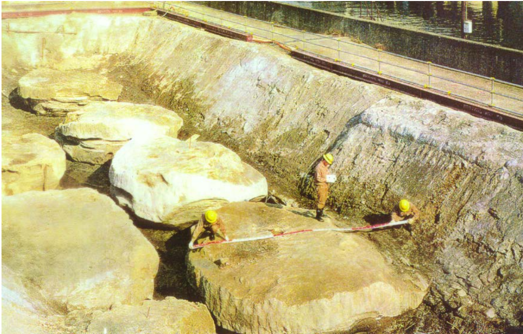
Fig. 1.5 The soil improvement columns developed by the super jet method
