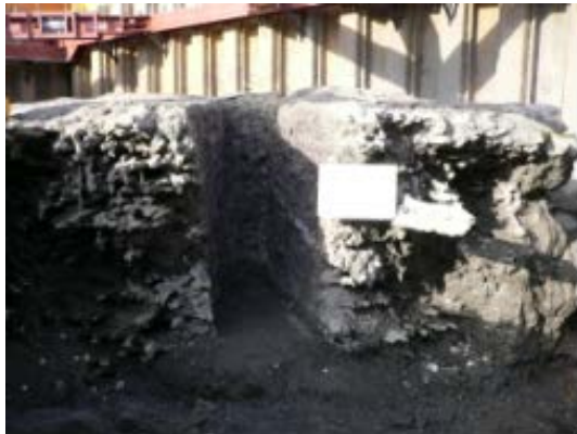
Fig. 4.4 JETCRETE column by the nozzle with flow conditioner with stepped lifting ( \phi 5.3\text{m} )
