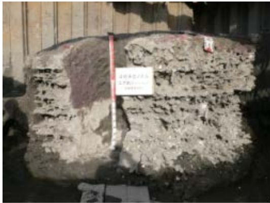
Fig. 4.3 JETCRETE column by normal nozzle ( \phi 4.0\text{m} )
