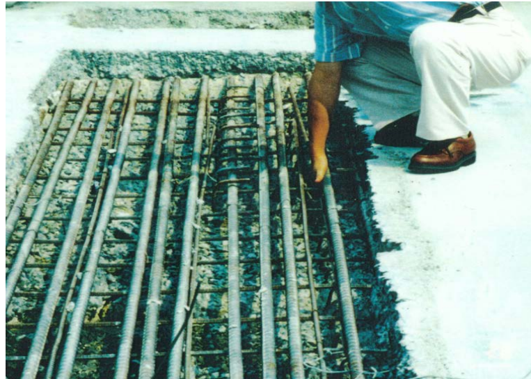
Fig. 1.10 Concrete cut by hydromilling method
