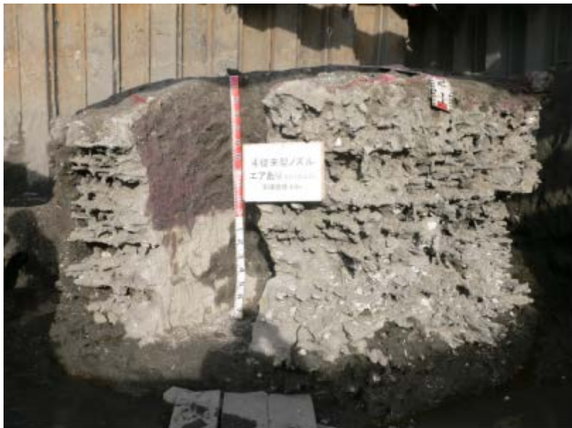
Fig. 4.20 Type 3 : JETCRETE column by normal nozzle with stepped rifting
