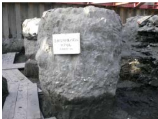
Fig. 4.9 Exposed JETCRETE column without air ( \phi 1.8\text{m} )
