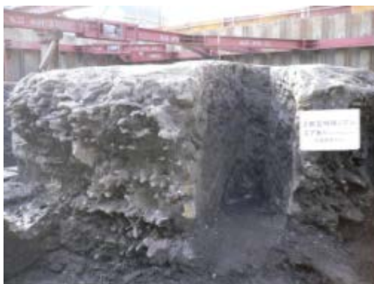
Fig. 4.5 JETCRETE column by the nozzle with flow conditioner with spiral lifting ( \phi 5.3\text{m} )
