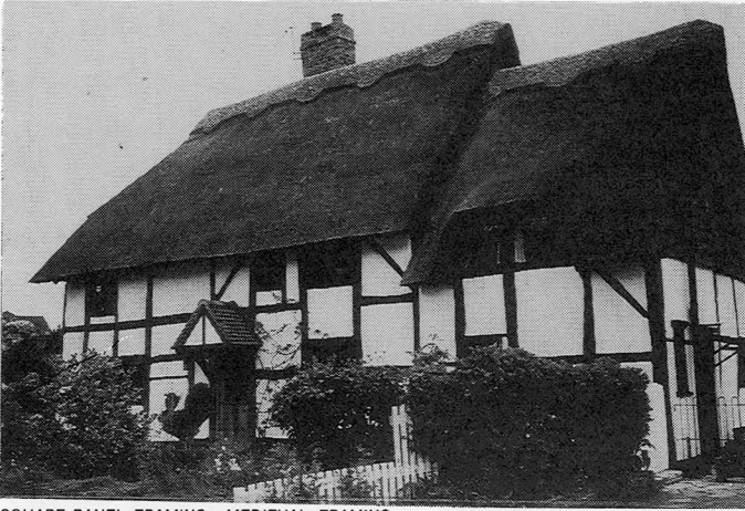
SQUARE PANEL FRAMING, MEDIEVAL FRAMING
