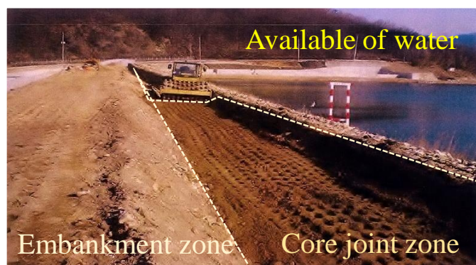
Figure 1.9 Heightening work for core heightening by inclined type (Site: Gyeryong reservoir, Gongju-si, Chungchungnamdo, South Korea, 2010)
