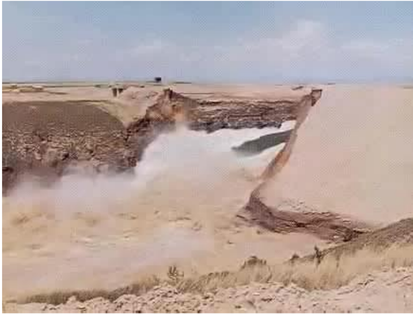
Figure 1.8 Teton Dam collapsed in Idaho, United States on June 6, 1976 (Piping through dam body) 7)
