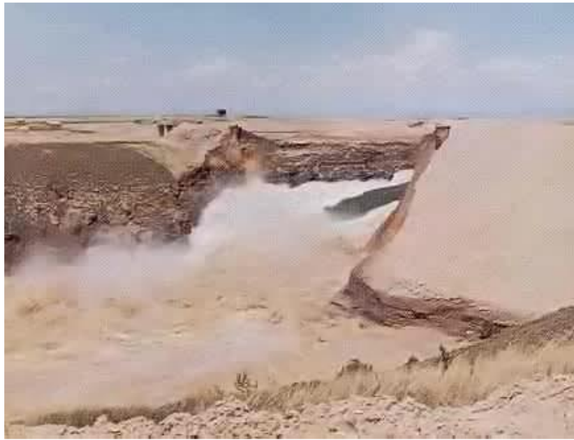
Figure 1.8 Teton Dam collapsed in Idaho, United States on June 6, 1976 (Piping thorough dam body) 7)
