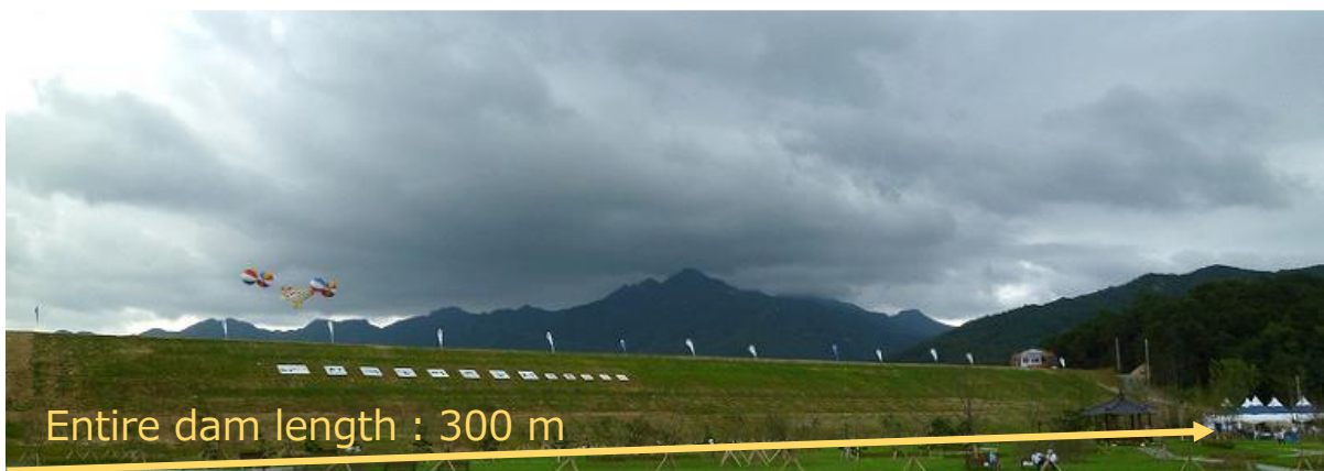
Figure 2.4 End of the dam in downstream-side (Gyeryong reservoir,2011.7)
