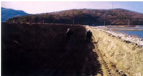
(a) Removed upper zone of the core
