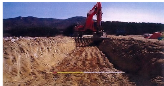
(b) Planed width of the heightened core: about 2m
