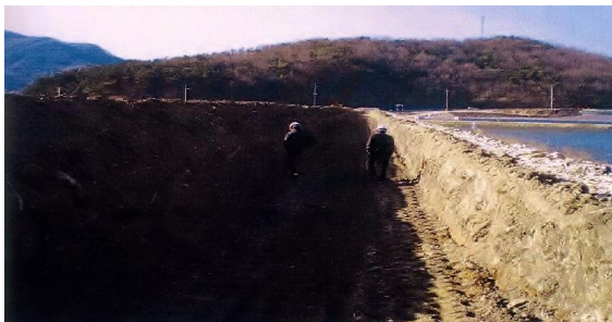
(a) Removed upper zone of the core
