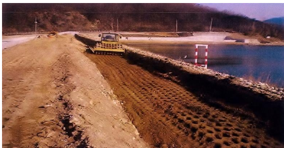
(c) Compaction work in core zone
