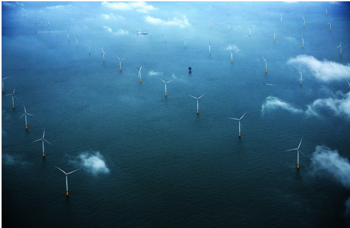
Figure 1-2 Overview of London Array
