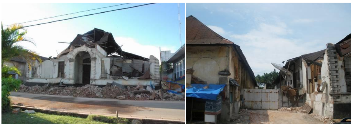
Fig.1.5 Debris clearing by the owner of cultural heritage building in Padang
