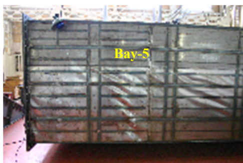
(e) Collapse of Hold-2 side shell
