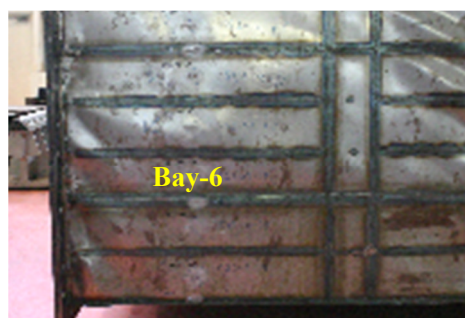
(b) Buckling of bilge corner
