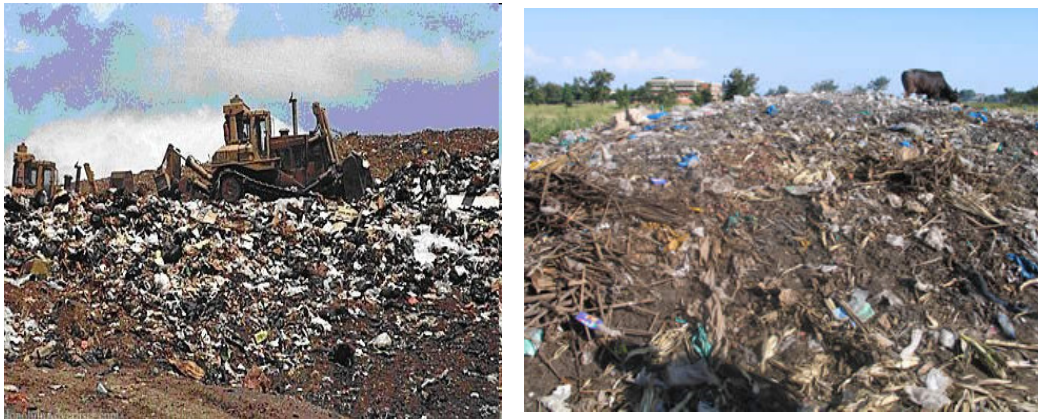
Figure 4.5 View of land fills
