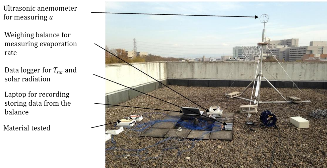
Figure 28. Actual set-up of outdoor experiment on October 29-30, 2014.
