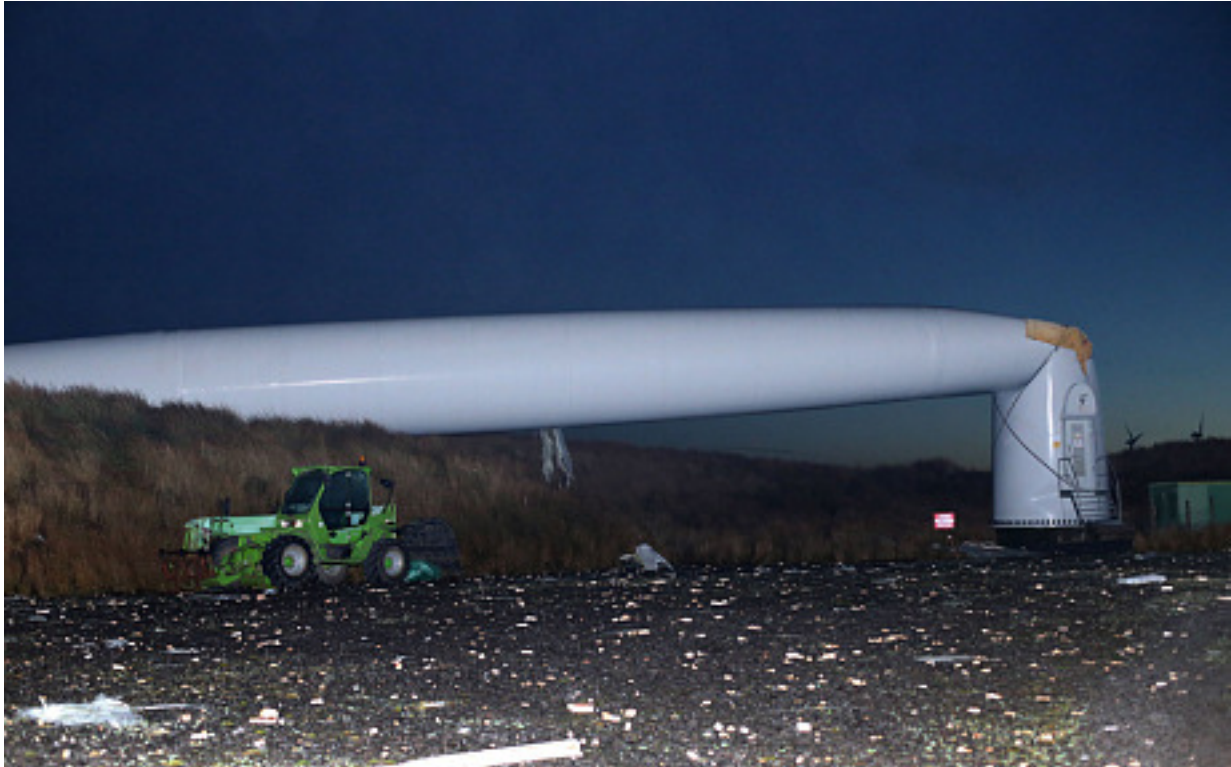
Figure 1.7 Northern Ireland wind turbine collapse. (Reproduced from Reference [25])
