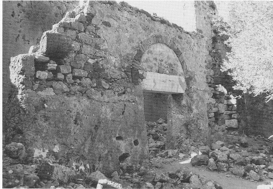
Fig. 44. Church III, Gemiler Ada. West wall.
