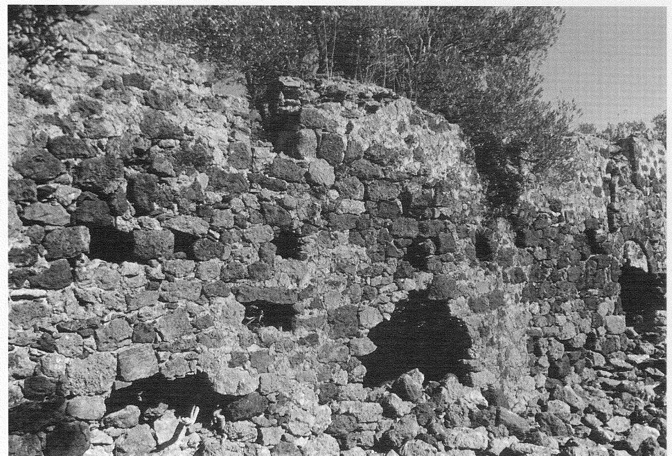
Fig. 59. Church IV, Gemiler Ada. South chapel.
