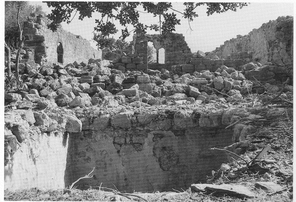
Fig. 66. Basilica on Karacaören Ada. Atrium.
