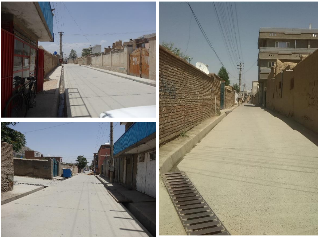
Figure 24. Street and houses condition in studied area of Afshar (Author's own picture)
