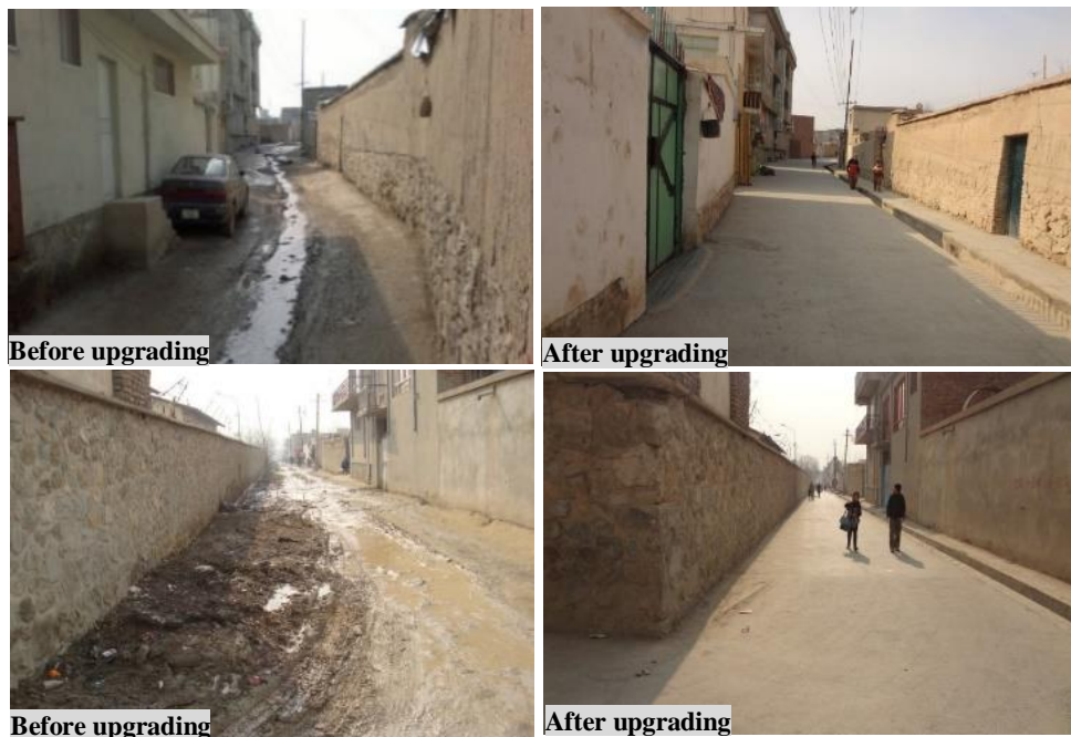
Figure 38. Streets and drainage improvement (Source: KMDP, 2016)
