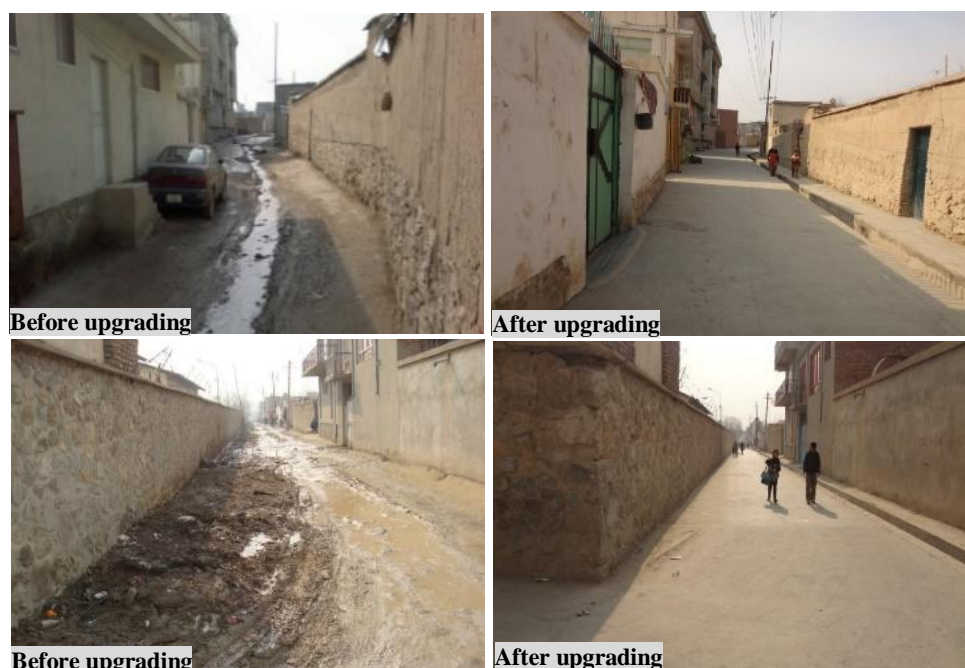
Figure 38. Streets and drainage improvement (Source: KMDP, 2016)
