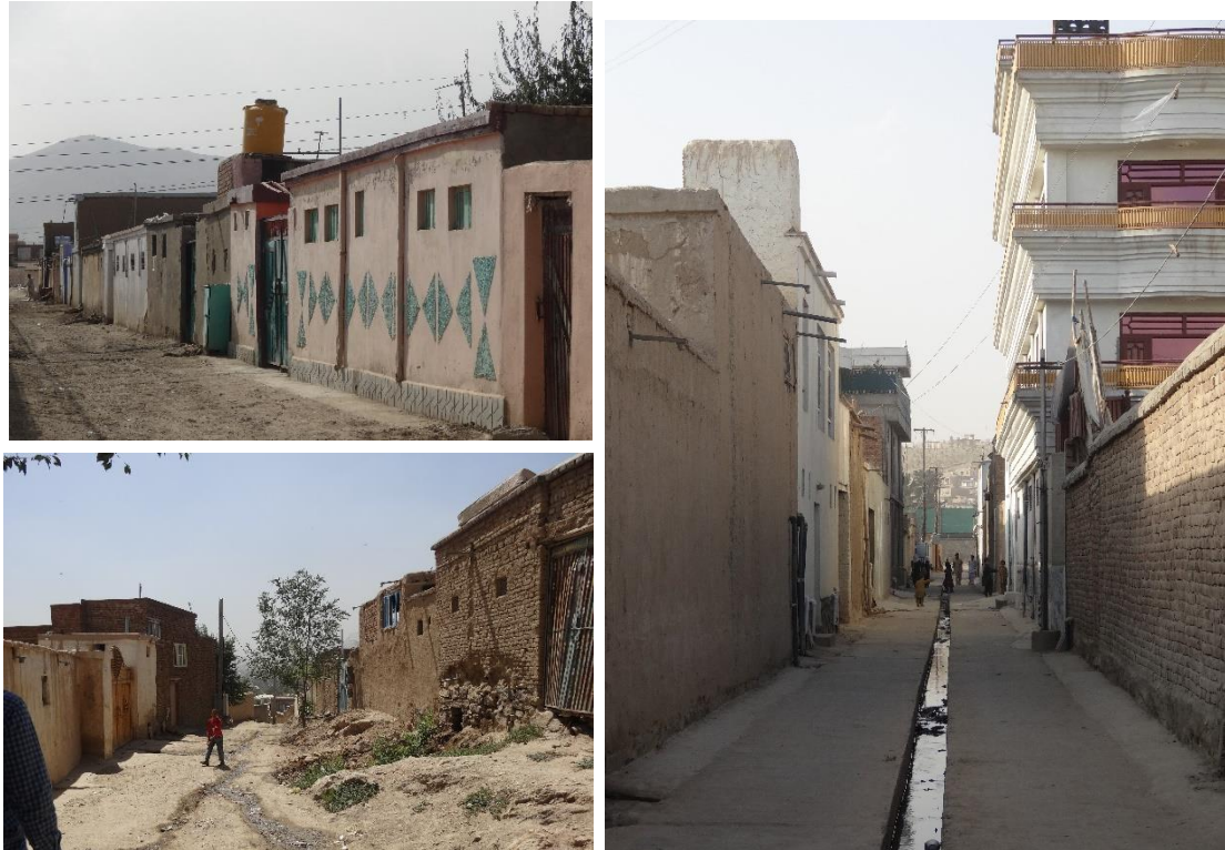
Figure 28. Physical condition of house in studied areas (Author’s own pictures)
