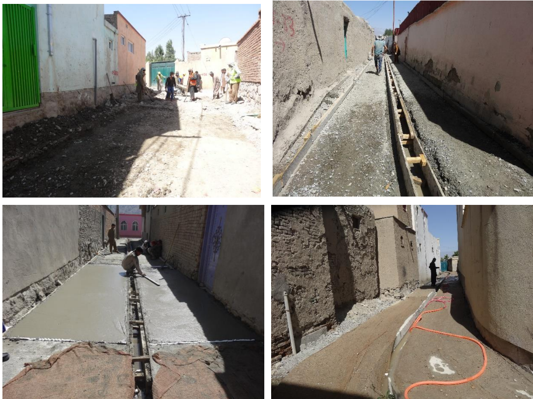
Figure 31. Process of streets and drainage improvement (Author's own pictures)
