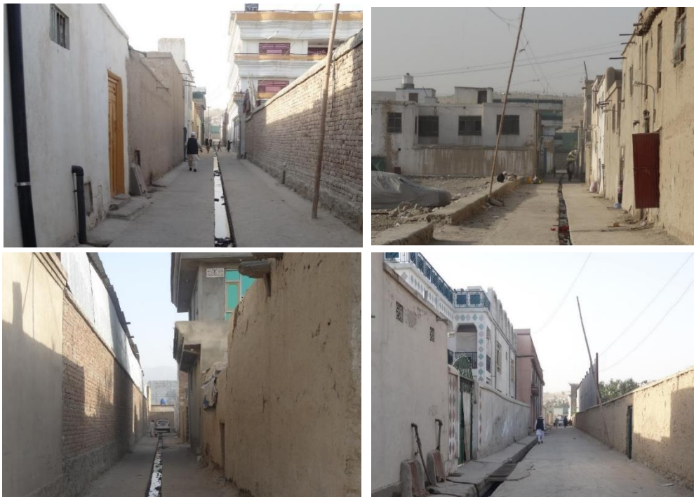
Figure 19. Street and houses condition in studied area of Shah Shahid (Author's own picture)
