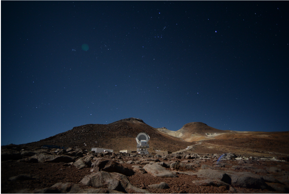
Figure 2.1.1: Picture of the observation site of the POLARBEAR experiment. The telescope in the center is the Huan Tran telescope (HTT) . There are four containers for operation and maintenance of the telescope.
