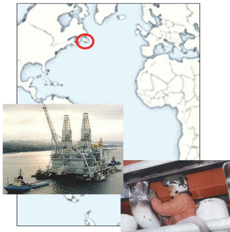
Fig.6.11 Application of developed FCW for low temperature service steel's SR part [Left] : Offshore structure in Hibernia, Canada [Right] : Application for pipe welding in Hibernia project
