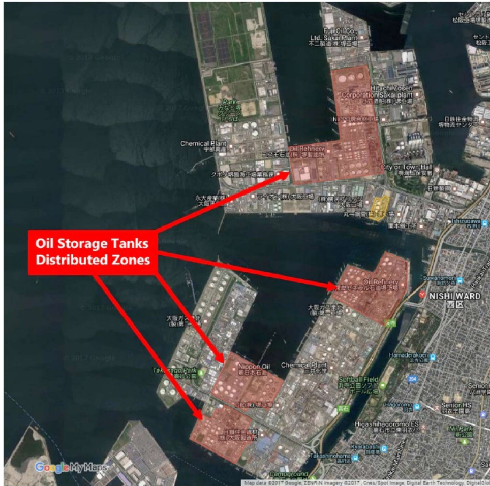
Fig. 5.4 Distribution of oil storage tanks in Sakai Senboku area
