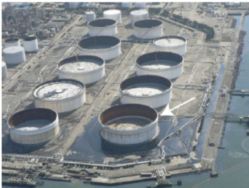
Fig. 1.1 Heavy oil spill out from conveying pipes in Sendai (FDMA)
