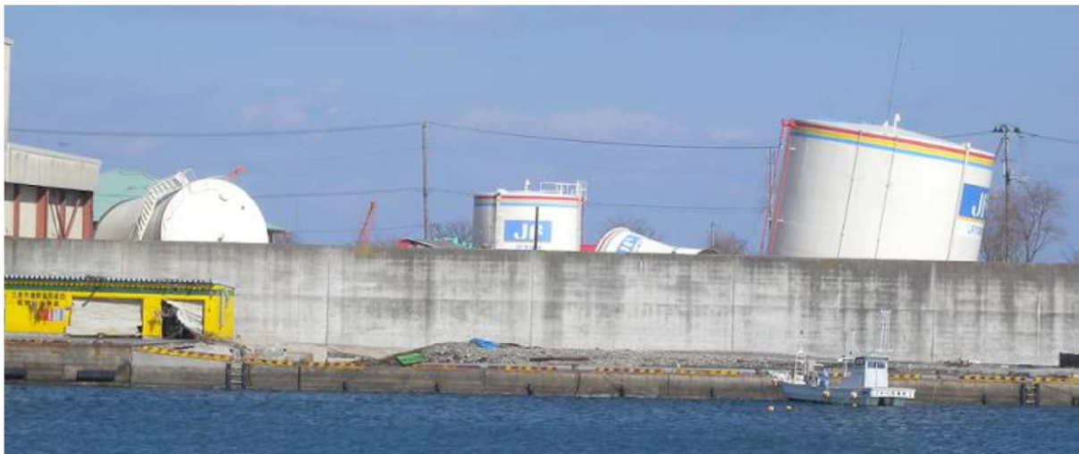
Fig. 2.1 Oil storage tanks damaged in the Port of Kuji after the tsunami of 2011 Great East Japan Earthquake
