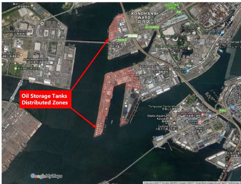
Fig. 5.3 Distribution of oil storage tanks in Osaka North Port area
