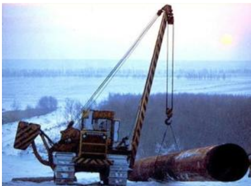
(c) Pipeline laying in extremely cold district.
