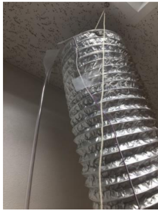
g) Measurement for exhaust air concentration h) Measurement for age of air
