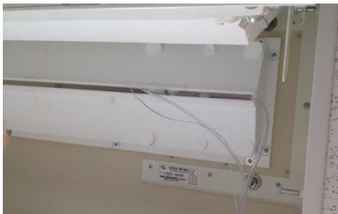
c) Measurement for supply air temperature
