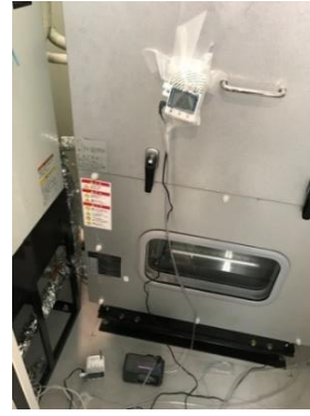
e) Measurement for supply air concentration f) Measurement for outdoor air concentration
