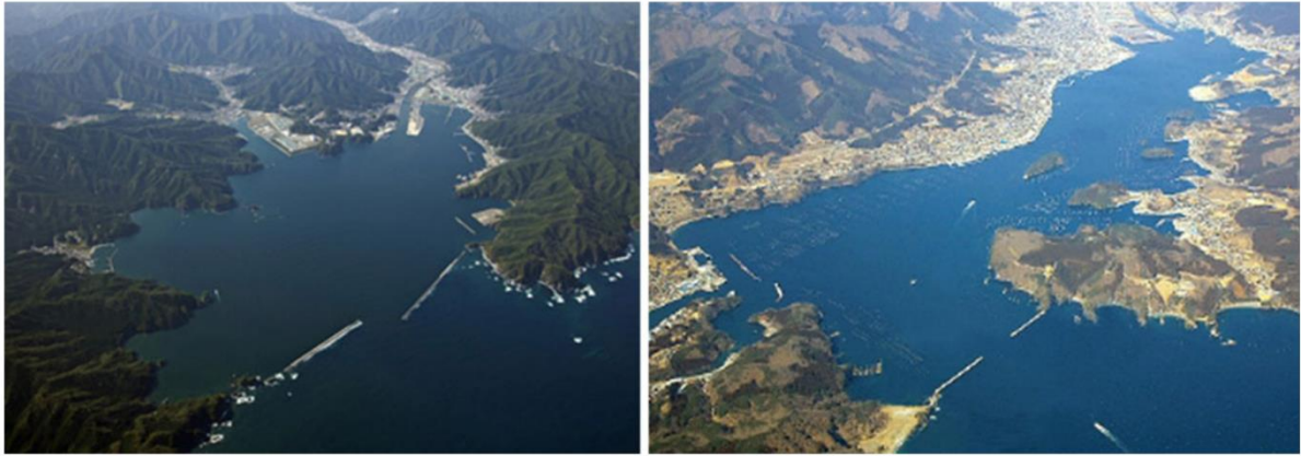
Fig. 2.1 Tsunami breakwaters in Kamaishi city and Ofunato city before the 2011 tsunami (Suppasri et al.)
