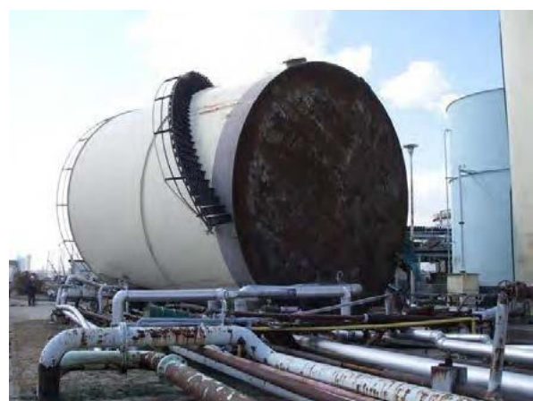
Fig. 1.2 Movement and tumbleness of large tanks (Fire Defense Research Centre, 2011)
