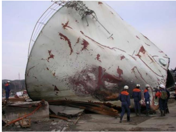
Fig. 1.1 Oil tank drifted and collapsed by tsunami (Fire Defense Research Centre, 2011)
