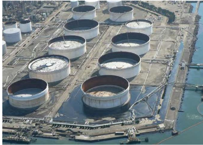
Fig. 1.3 Oil spill occurred from a tank, with the leaked oil inside and outside the dyke wall (Fire Defense Research Centre, 2011)
