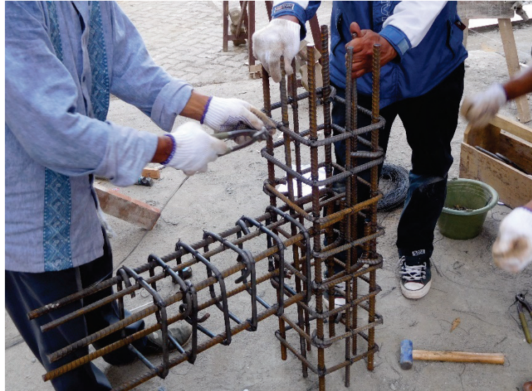
Figure 2.6 Rebar fabrication by local workers in the workshop
