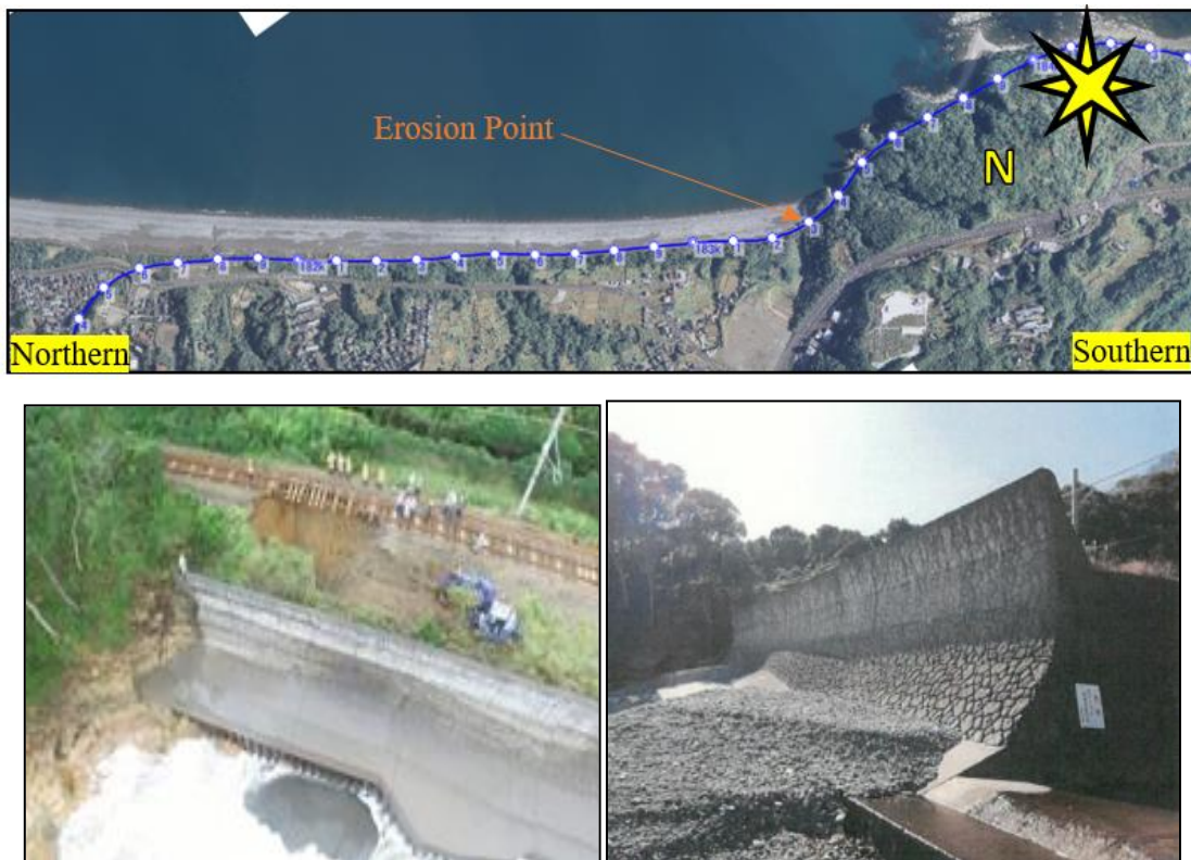
Figure 2.1 Location of erosion as a result of high wave generated by typhoons
