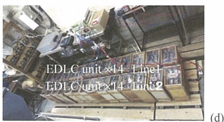
図10 大容量EDLCの静電容量不揃いとPC動作 Fig.10 Operation of overvoltage protection circuit in large-capacity EDLC connected in series [(a) Not adjust the capacitance balance of EDLCs connected in series, (b) Photograph of test circuit of (a), (c) Adjust the capacitance balance of EDLCs connected in series (d) Photograph of test circuit of (c)]
