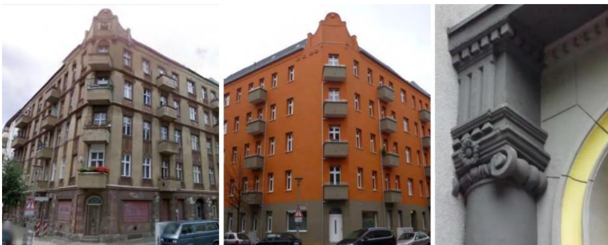
Figure 59: Historical building heat insulated in Berlin. Left: the original façade; Middle: insulated façade; Right: the insulation damaging the historical decoration (Budapest University of Technology and Economics, Faculty of Architecture, 2016)
