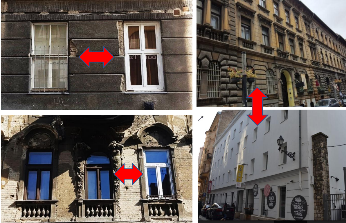
Figure 62: Individual, unprofessional window exchange or insulation causes uneven fa ades and loss of character. Pictures are Courtesy of Attila ZSOLDOS BSc Architect
