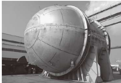
Fig. 6.1 Liquefied hydrogen 1000m 3 test tank[103].
