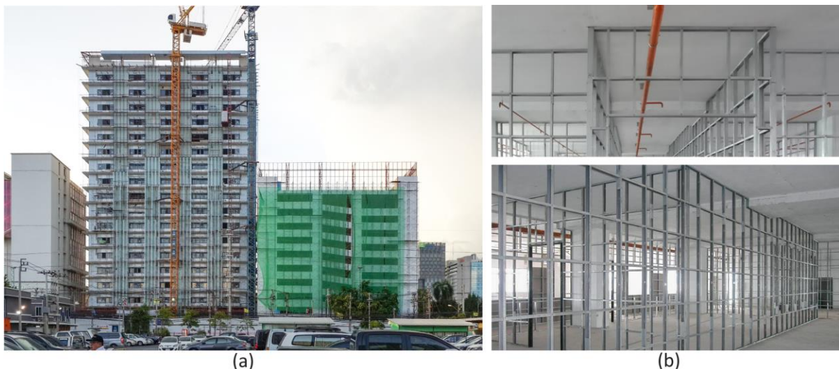
Figure 5.14 (a) Chulapat 14 building. (b) Interiors of the fifth and the sixth floors during construction.
