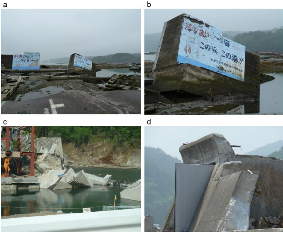
Figure 1.7. Seawall damage observed during the 2011 tsunami disaster: (a) damage to seawall and quay at Minamisanriku; (b) close-up of sea wall block at Minamisanriku showing no inter linkages; (c) recovery work on the seawall at MiyakoBay; and (d) remaining seawall buttress at Tarō.
