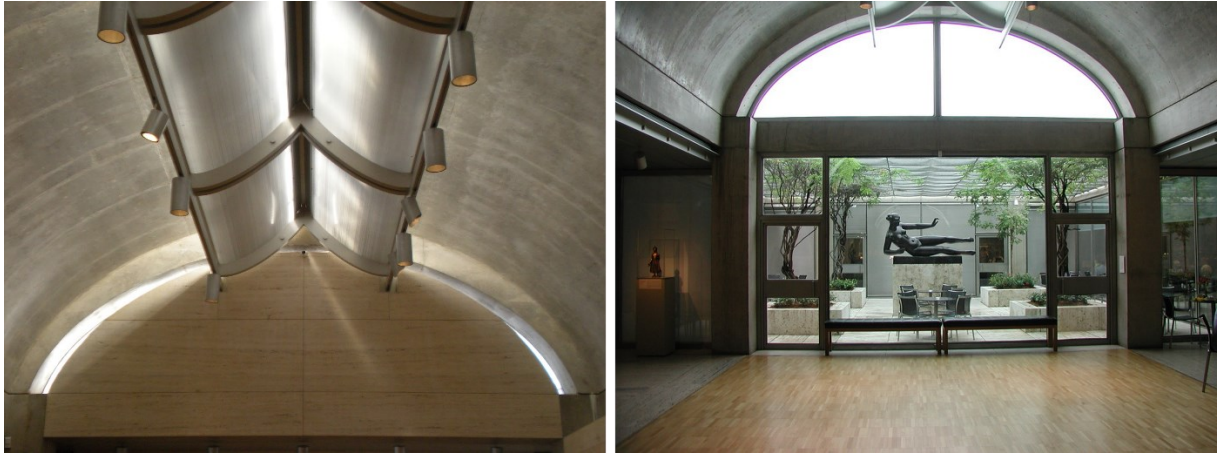
Figure 48: (Left) Close-up for the reflector and vault slit (right) Main courtyard (Kimbell Art Museum 2020).
