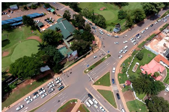
Figure 4-5: One of the upgraded intersections
