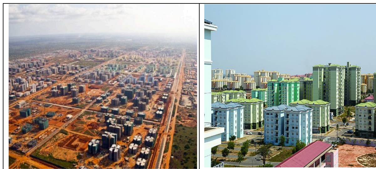
Figure 3.4 Kilamba Housing Project a) During construction and b) after construction (source Cain, JA) - Kilamba New City in Luanda, China's Largest Housing Project in Africa Source: Allan Cain, 2014
