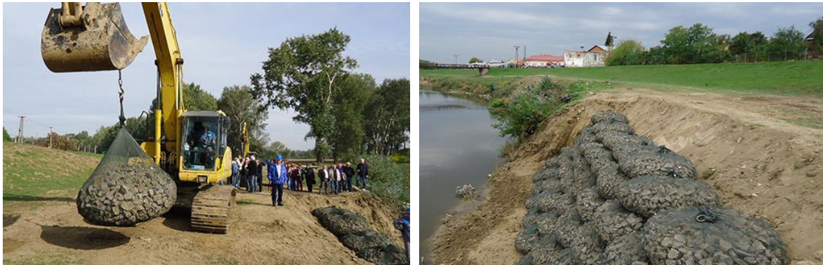
Figure 1. 6 FU application for river bank protection (one of Kyowa's Projects)
